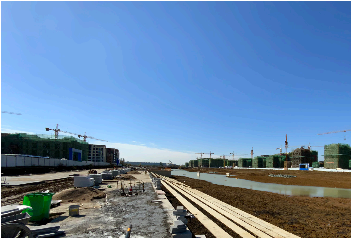
under construction, picture taken in 2021.
